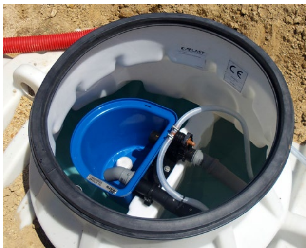
Figure 1: Left: Construction of Modified Septic Tank (Aerated Fixed Bed Reactor). Right: Load-controlled SBR (PUROO).
