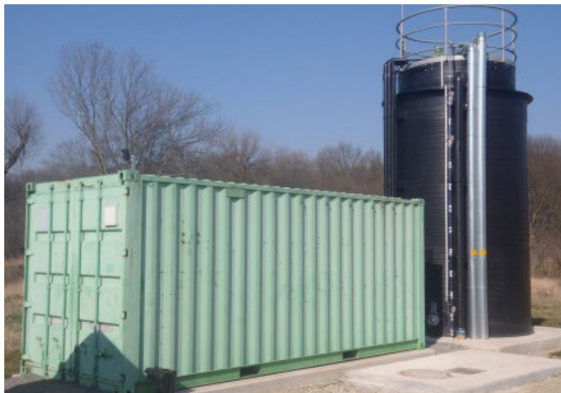
Figure 1: Left: A dosing station (22 m 3 ) and a container with a mixing tank inside. Right: The distribution system for loading and O&M of the DWWT-technologies at the BDZ.
