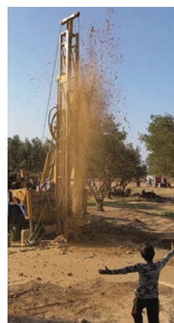
Figure 1: Left: Groundwater fountain by rotary drilling from borehole in Deir Alla. Right: Potential for Managed aquifer recharge in the Jordan Valley.
