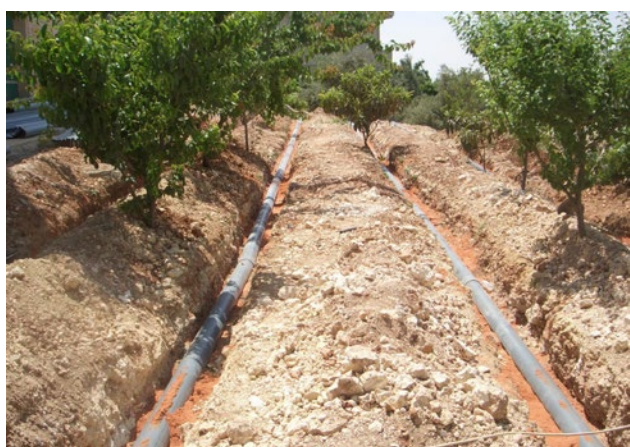
Figure 2: Left: Subsurface irrigation system for treated wastewater. Right: Wastewater treatment plant at Princess Rahmeh College (Aerated Horizontal Filter).
